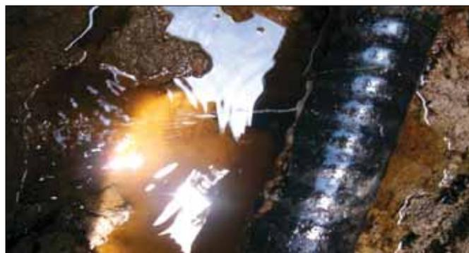
Fig. 10: Typical sheath leak.
